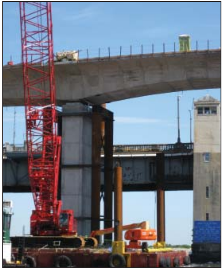
This Johnny On The Spot portable restroom is located on the bridge deck.
